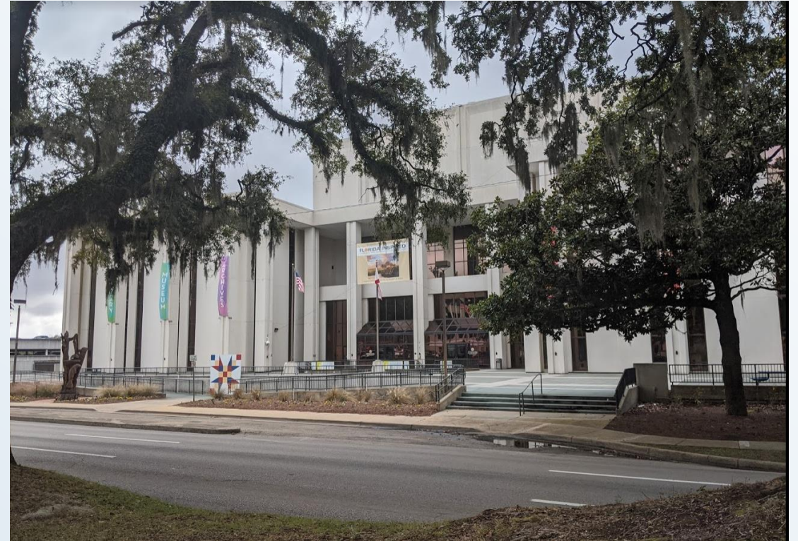
R.A. Gray Building, Tallahassee, FL.
